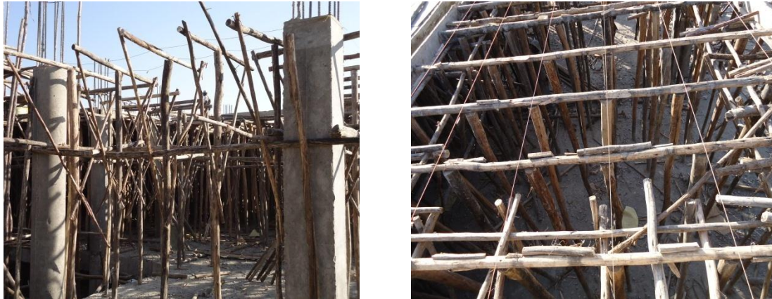
Figure 3.2 Formwork Preparation
